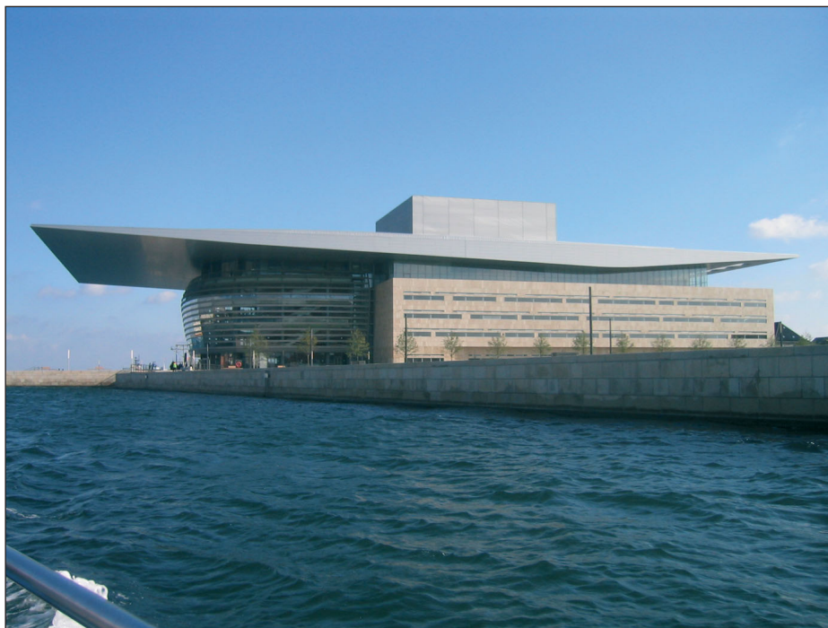
Fig. 1: Opera House, Copenhagen
